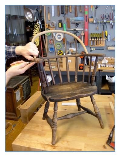
After gluing the hoop in place, it was treated with a weak chemical that reacts with the natural tannins in the oak and ages it a century in less then an hour.
